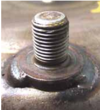
FIG 1. This stud has threads the full length of the stud.
